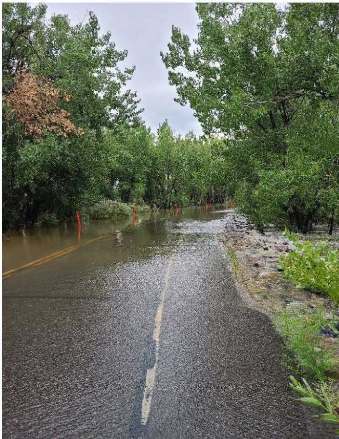
Storm Photo - Cherry Creek at Lake View Drive General Assessments
